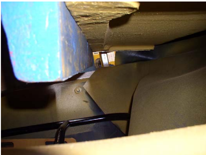
13: After lowered, check no gap exists at the bottom.
