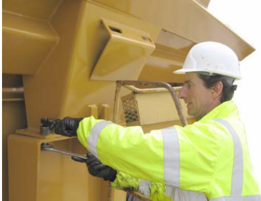
13: Fit & tighten bolts at hopper leg/ chassis. (Both sides.)
