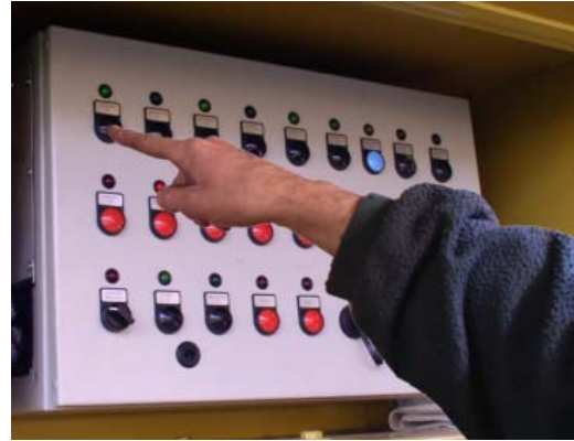
2: Press button INTERLOCK ON.
