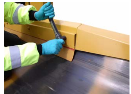
3: Refit clamp fixing screws.
