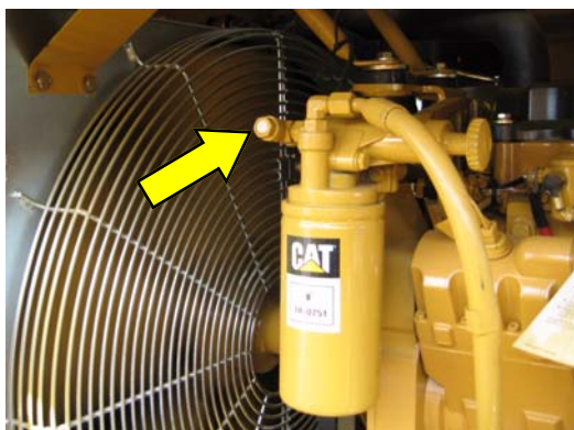
1: Loosen bleed screw on fuel filter. (EN1001)
