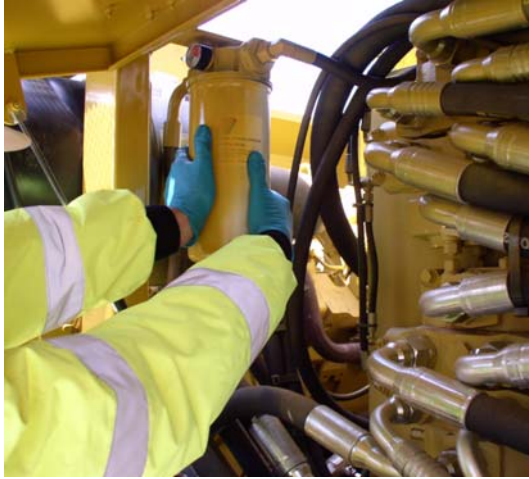
1: Replacing hydraulic water trap. (EN1401 & EN1404)
